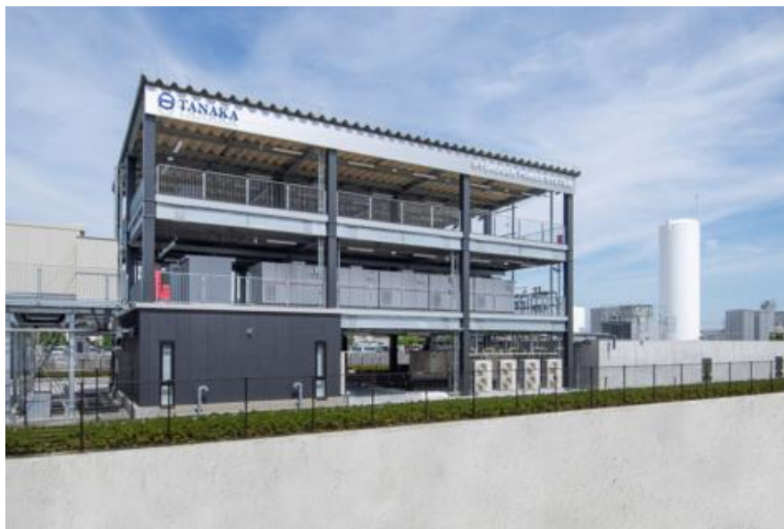
<TANAKA Shonan Fuel Cell Power Plant: Fuel Cell Power Generation Facility "TANAKA H2 Nexus">
