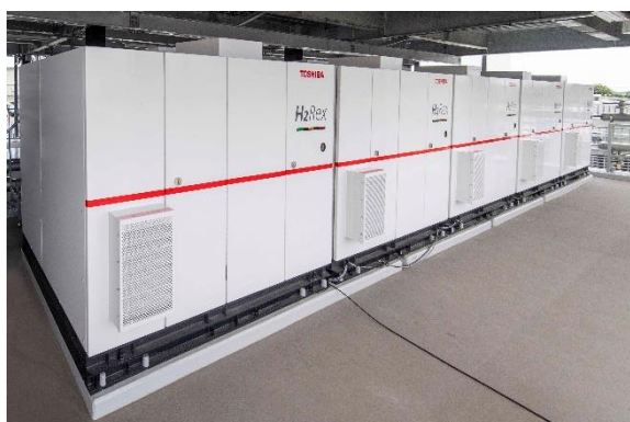
Photograph: Toshiba's "H 2 Rex™" Pure Hydrogen Fuel Cell System
